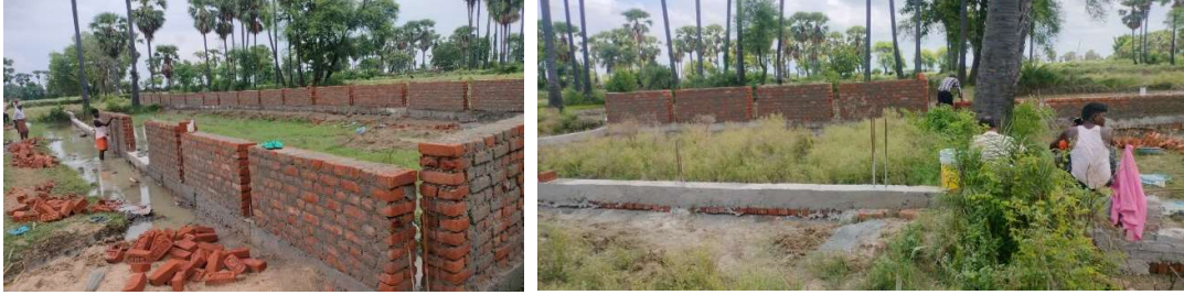
Making the boundary wall around the land purchased by the school.
