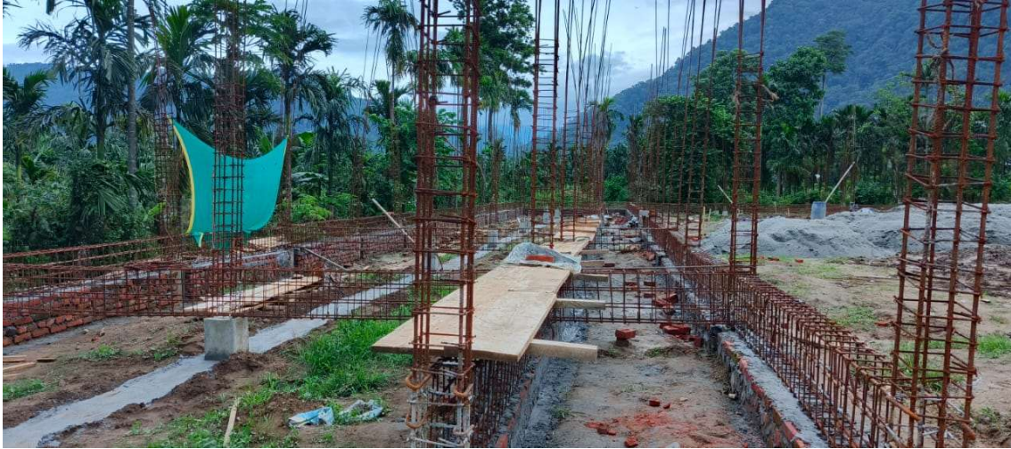
Foundation work for the classrooms
