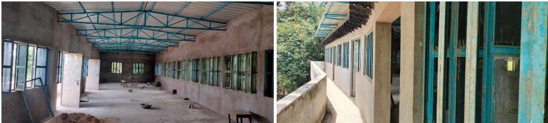
Renovation of the classroom and hall for the students
