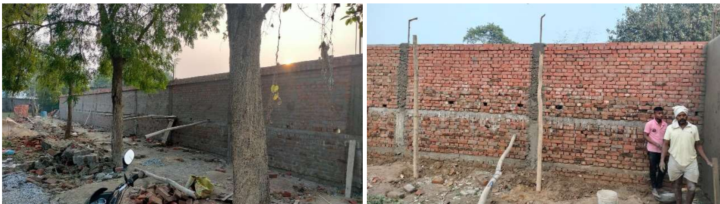
Constuction of the boundary wall at the school of Sarnath.
