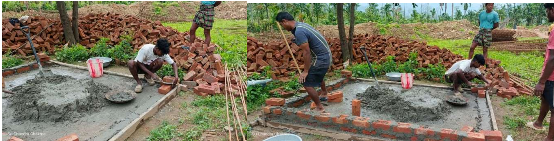
Construction of the tank for the pit
